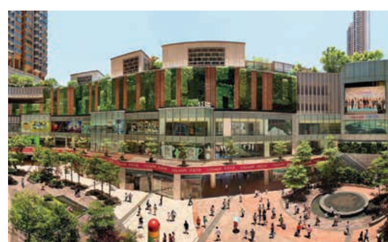
Citywalk & Citywalk 2 received the Gold Award at the Inaugural Skyrise Greenery Awards by the Development Bureau. The project is also rated Platinum by HK-BEAM Society
