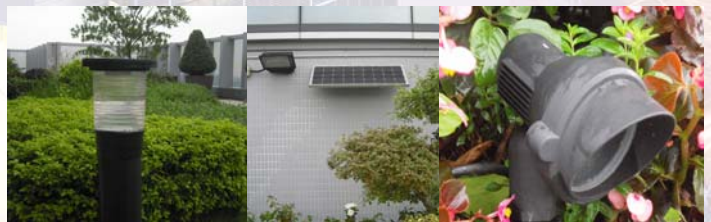
Solar Panel and Lighting are installed at Roof Garden
