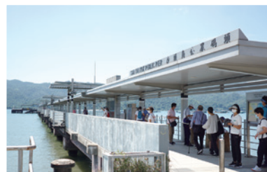
Longest Pier in Hong Kong: Sha Tau Kok Pier
