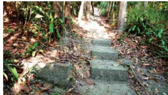
**Figure 74:** Concrete steps found on the hillside below the store room. They go down to the old path to the engine room. These steps were possibly built by the military to connect the store room and engine room (photo by author in 2019).
