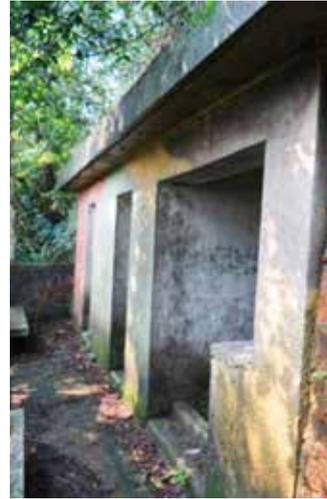
**Figure 13:** An early military toilet at Pinewood Battery. The wash stand is in front and the two toilet rooms are in the back. Note the camouflage painted on its wall (photo by author, 2000s).
