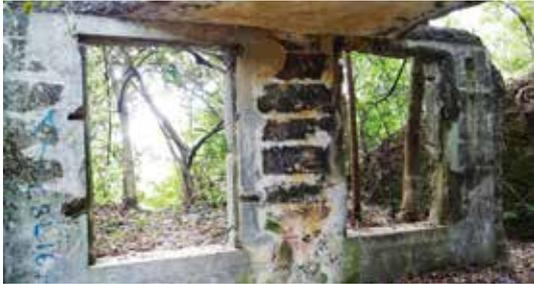
**Figure 69:** Inside of the front wall and window of the store room. The square hole at the top right is for ventilation (photo by author in 2014).
