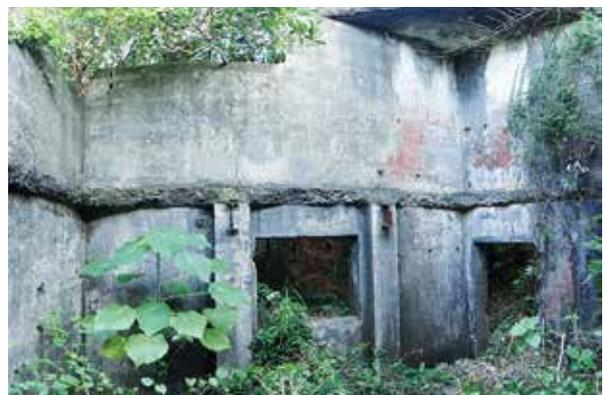
Figure 46: The right interior of the Ping Tok Hang Shan AOP. Its design was the same as that of the Tai Leng Tung AOP. The roof and upper floor of this AOP were demolished after the war (photo by author in 2016).
