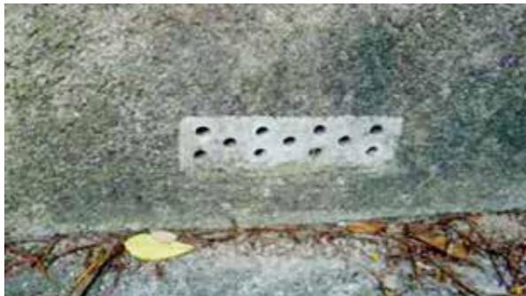
**Figure 12:** Ventilation holes along the front wall of the shelter (photo by author, 2007).
