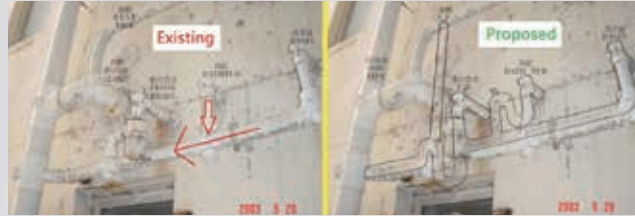
2003 - Drainage Improvement at Amoy Garden
