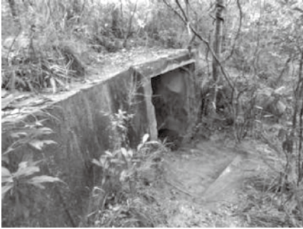
Figure 60: An entrance to tunnel near the shelters. Half of this entrance was blocked by a concrete wall before. This may be an emergency exit for the tunnel. Note a concrete step outside the entrance (Photo by author in 2010).
