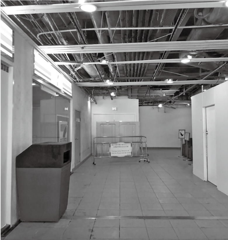
Figure 23: View from outside the toilet
