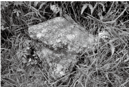
Figure 9: GDL marker stone below PB125 at Shatin Pass. Most of the
