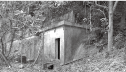
Figure 34: HQ shelters re-opened in 2013. Note the drain pipe fallen on ground which was still intact in 2000 (Photo by author in 2013).
