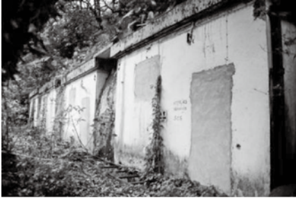
Figure 33: Four sealed HQ shelters. Note the building structure registration number marked on the shelter. This number is normally for temporary squatter buildings. Many wartime military structures were considered squatter buildings by the government and demolished (Photo by author in 2000s).
