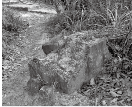
Figure 13: GDL marker stone at Shatin Pass damaged circa 1990 still with its top surface. (Photo taken by the author in 2011.)
