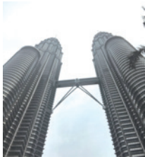
Fig. 13 A two-hinge arch supporting the Skybridge 6
