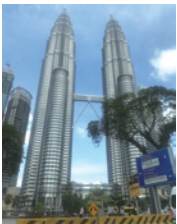
Fig. 12 Petronas Twin Towers with a Skybridge
